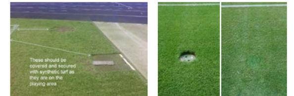
Fig. 28. Access and service boxes within the safety zone around the field of play.
