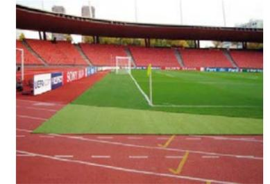
Fig. 27. Extension of turf perimeter around the field of play using high-quality artificial turf.
