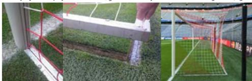
Fig. 24. Goal frames recessed into the ground.
