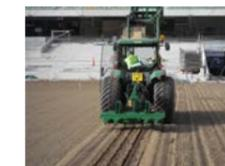
Fig. 7. Installing undersoil heating pipes through the profile.
